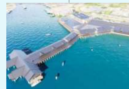
Redevelopment of Sunway Pier
