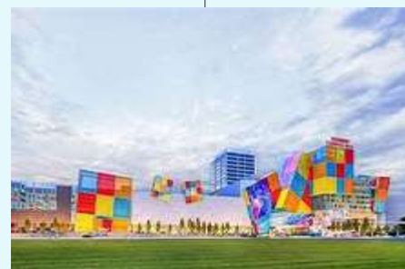
Sunway Carnival Mall Existing Wing
